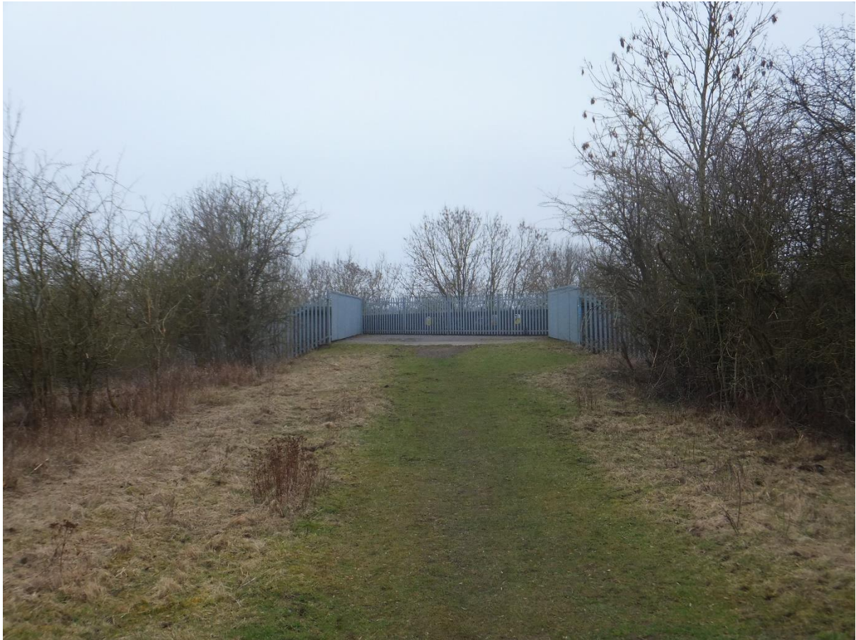
Figure 4 Looking south from the GCR trackbed at the furthest southern extent of this portion before a missing bridge is reached (SP 5179 7644).
