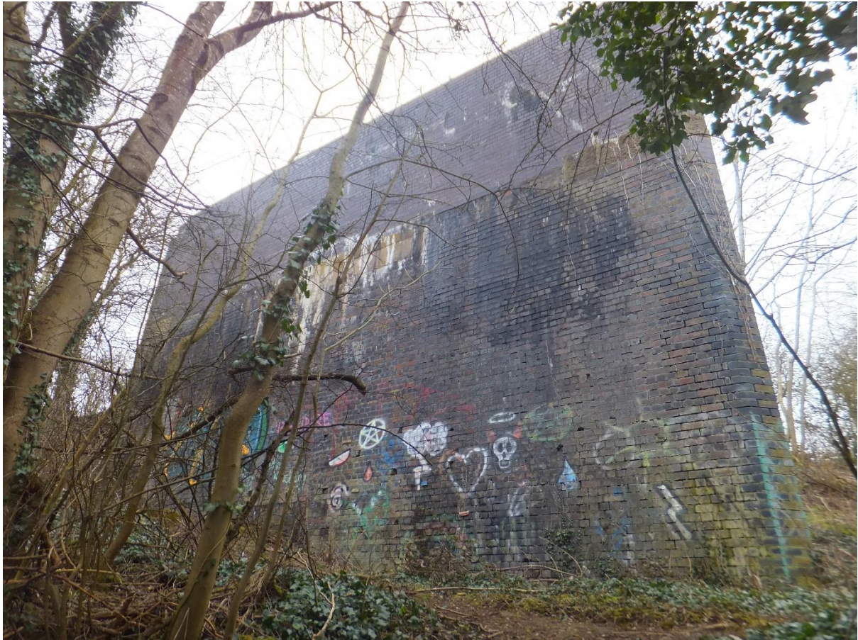
Figure 3 Looking north at the end of the walkway carrying the GCR trackbed. A missing bridge would have carried the railway south here across the Oxford Canal (SP 5179 7644).
