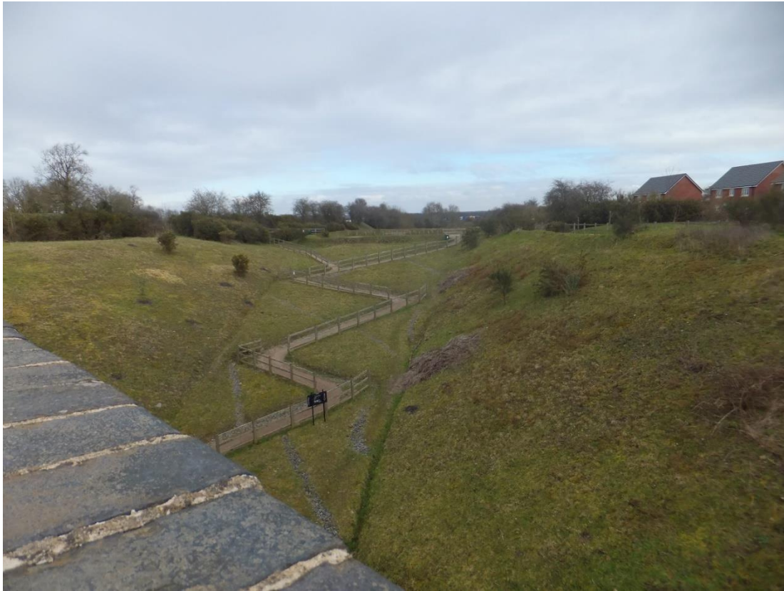
Figure 13 Looking northeast from the top of the Newton Lane bridge at the zig-zag footway up to the top of the filled in section of cutting (SP 5300 7857).
