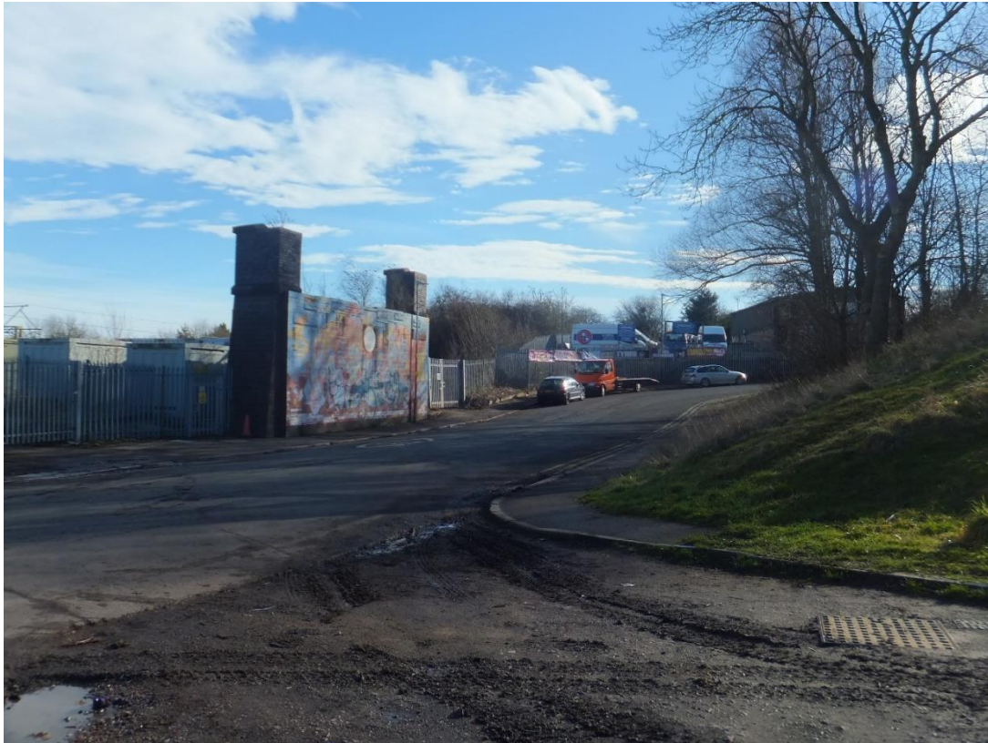
Figure 11 Remains of the bridge taking the GCR across Abbey Street just before it reaches the West Coast Main Line (SP 5161 7570).
