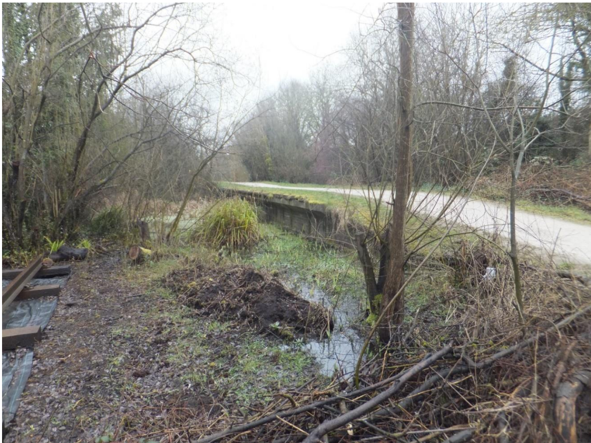
Figure 9 A closer look at the platform at the former Rugby Central station. Looking north from the trackbed (SP 5139 7447).
