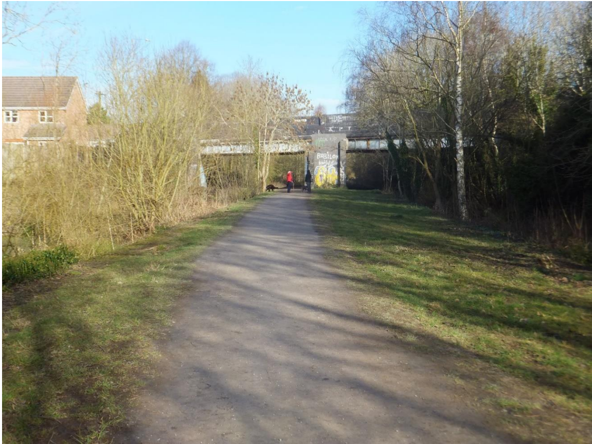
Figure 8 Looking north towards Hillmorton Road bridge from the platform at Rugby Central station (SP 5137 7461).
