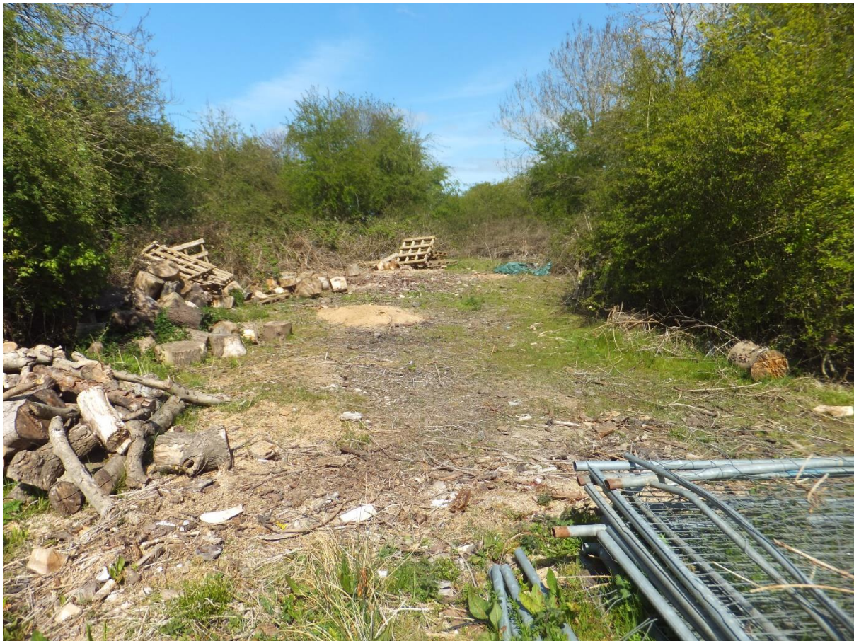
Figure 7 Looking north along the trackbed at a small open section south of the water-filled area (SP 5222 6296).
