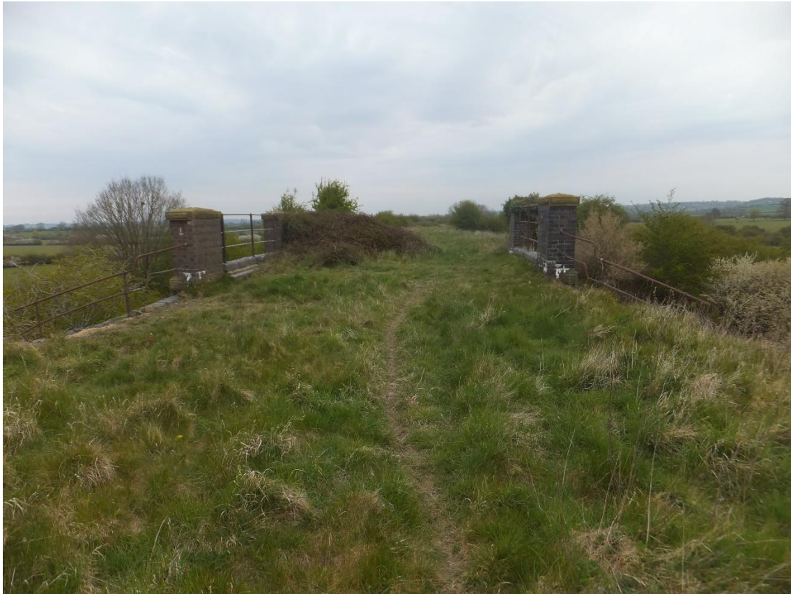
Figure 21 Looking north along the embanked trackbed north of the Oxford Canal near Braunston, just south of a short bridge where there is an access track below (SP 5243 6567).
