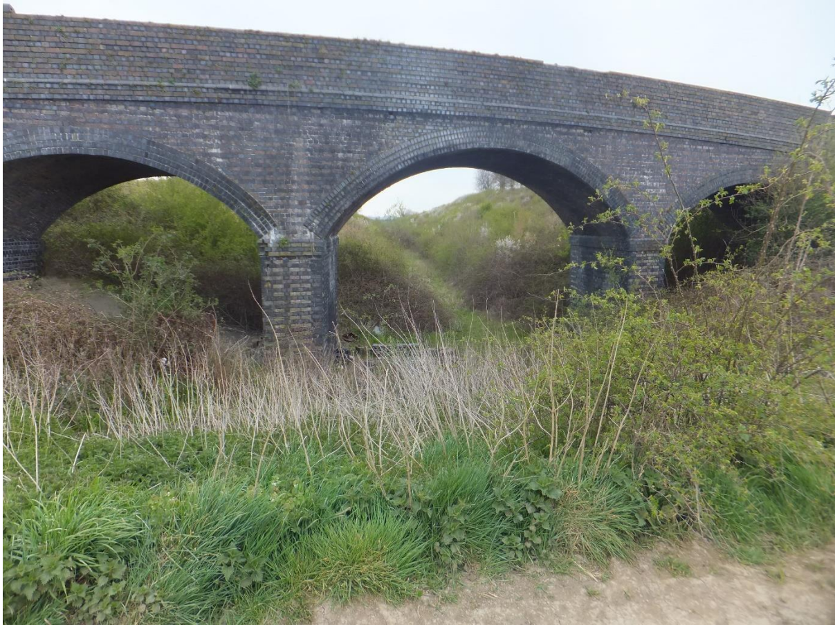
Figure 13 Looking south at the triple-arch bridge over the trackbed at SP 5244 6434.
