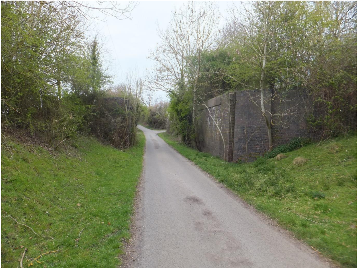
Figure 18 Looking south-west along the gated road between Wolfhamcote and Flecknoe where the GCR would have crossed on a missing bridge (SP 5244 6506).
