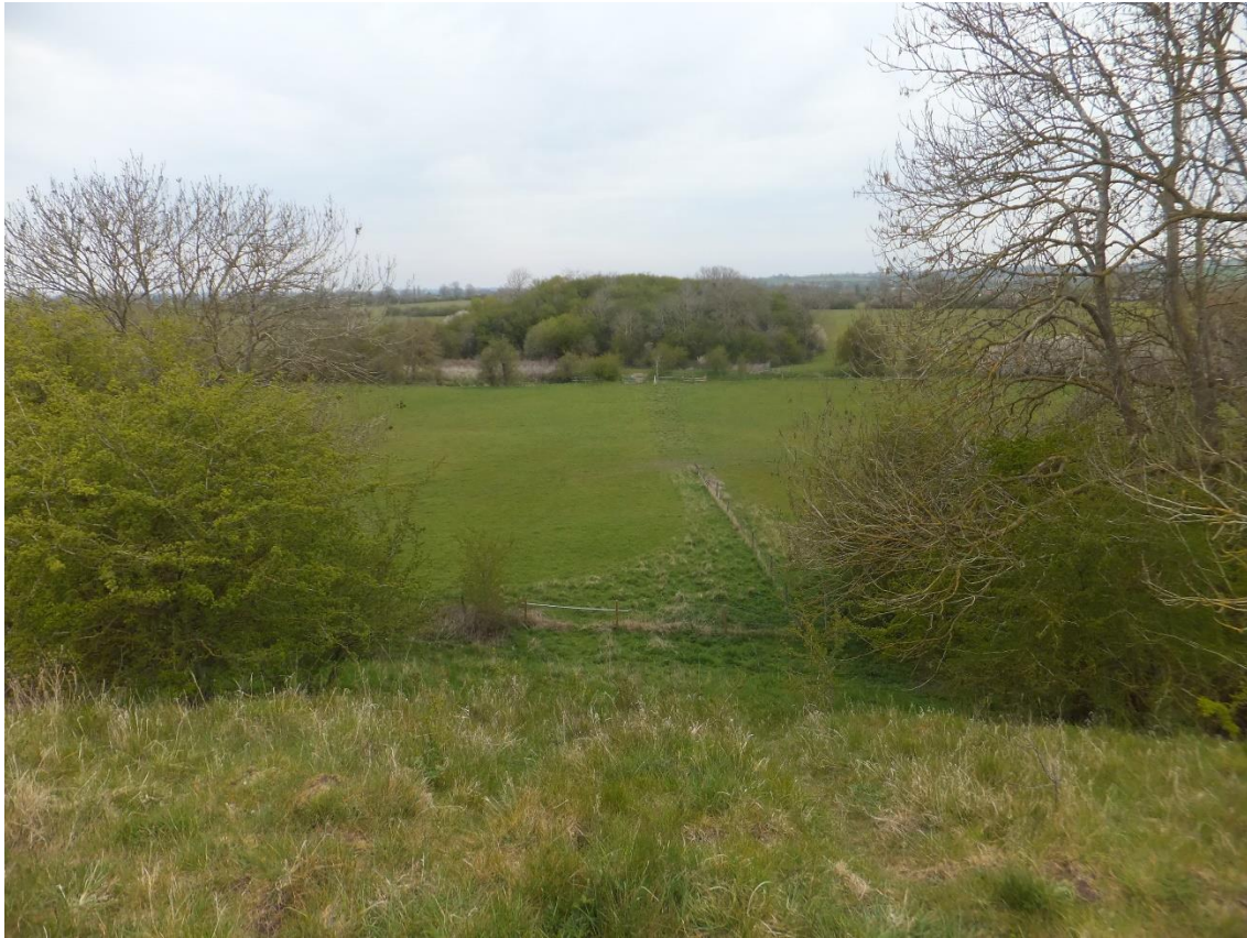
Figure 22 Looking north at the end of the embankment before a gap is reached at SP 5242 6596. The River Leam flows east-west just before the trees on the far side.
