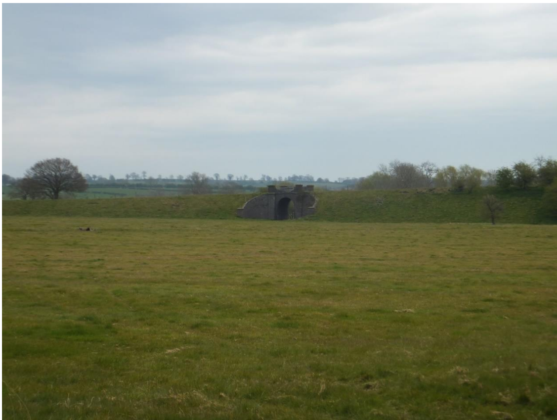
Figure 24 Looking north-east towards an access bridge within the GCR embankment south of Willoughby (bridge at roughly SP 5242 6655).
