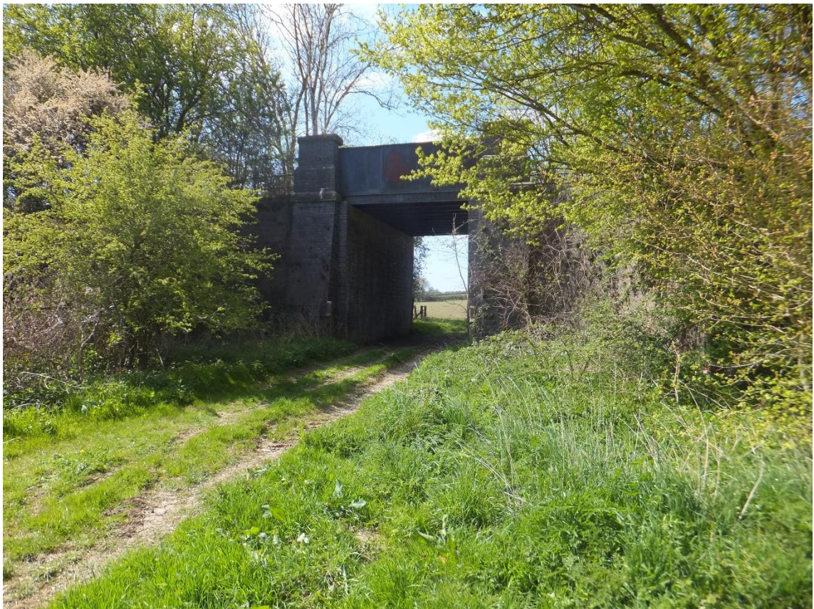
Figure 4 Looking west at the access bridge carrying the GCR trackbed (SP 5214 6279).
