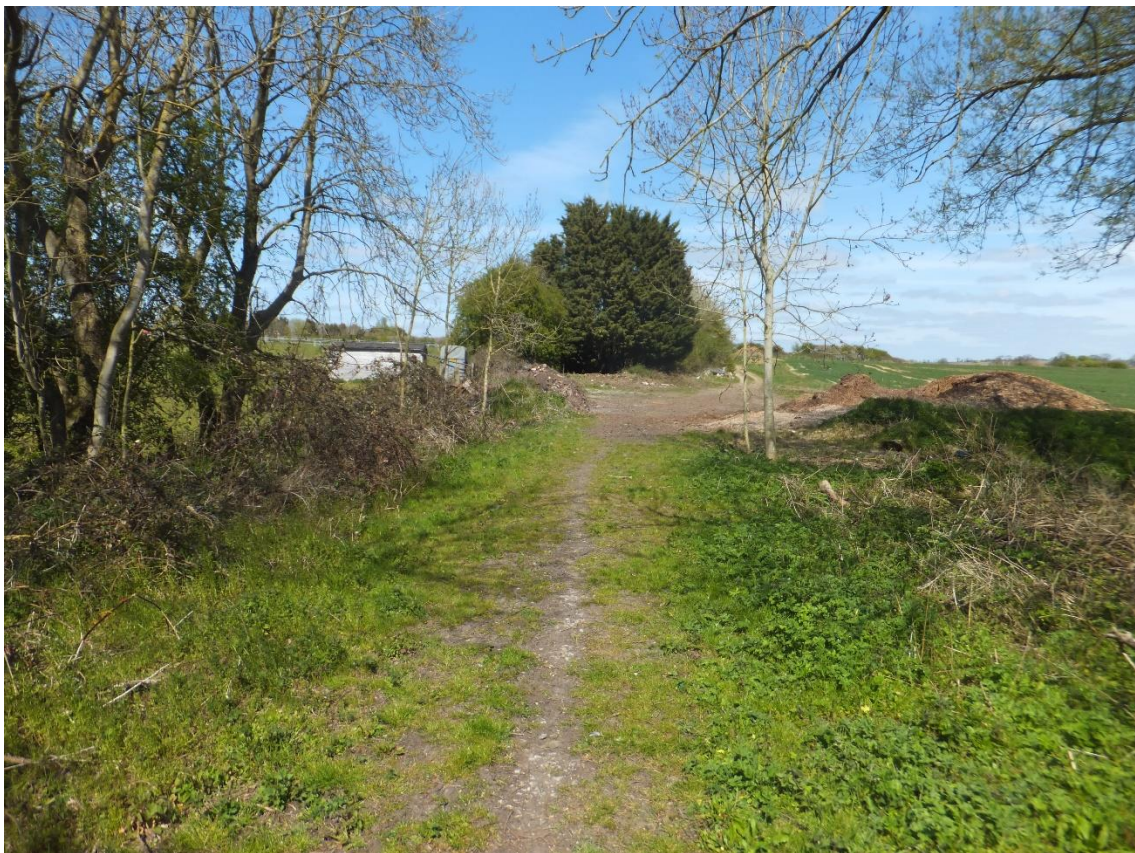
Figure 6 Looking north along the trackbed at the northernmost extent of a walkable section south-east of Flecknoe (SP 5218 6290).
