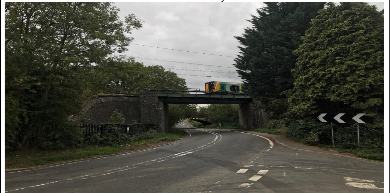
Caption Below: A local West Coast Main Line train approaches Rugby on the Northampton Loop Line which with the fast lines via Blisworth, fans out south of Rugby. Picture taken from the A428 Crick Road, Rugby by Mr Stephen Byatt 2018. The Great Central link line would have to connect from Willoughby area on the traditional Great Central corridor to these lines somehow via Barby.
